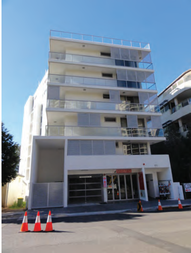
Recent development 111 Wigram Street - 6 storeys street wall and up to 9 storeys above
