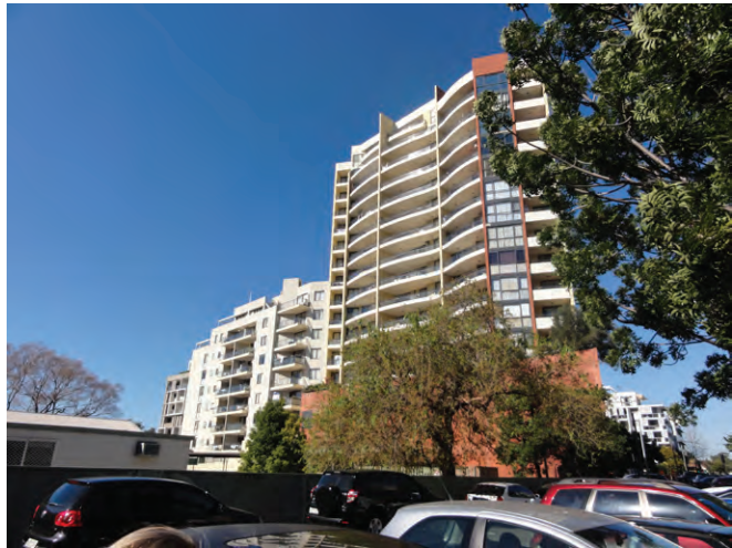
Buildings fronting Hassall Street seen from the northern side of the subject site
