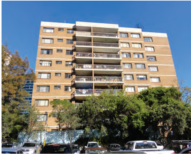
9 storey residential building on the south-western corner of the site
