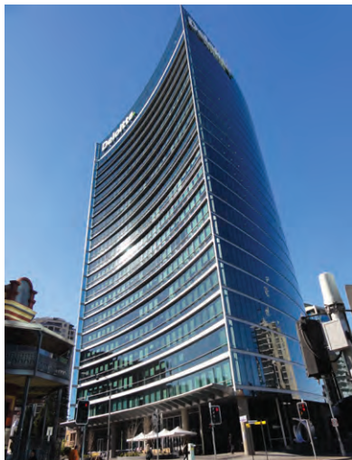
Deloitte Building at 60 Hassall Street
