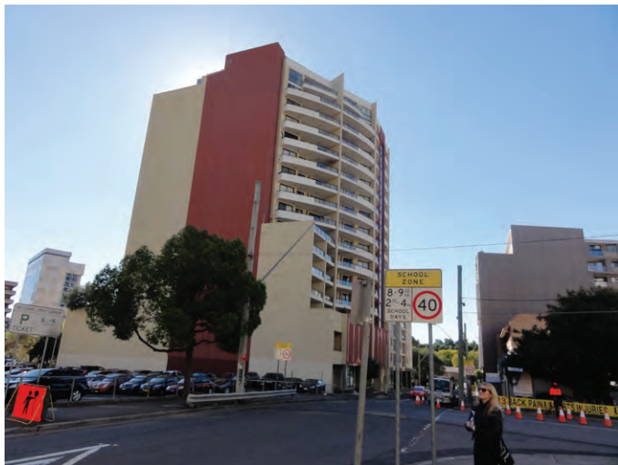
26-30 Hassall Street - 17 storey building to the east of subject site presenting a blank wall toward the site
