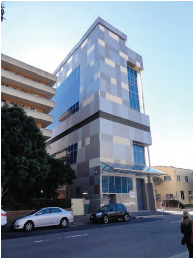
Infrastructure building (9-10 storeys)
