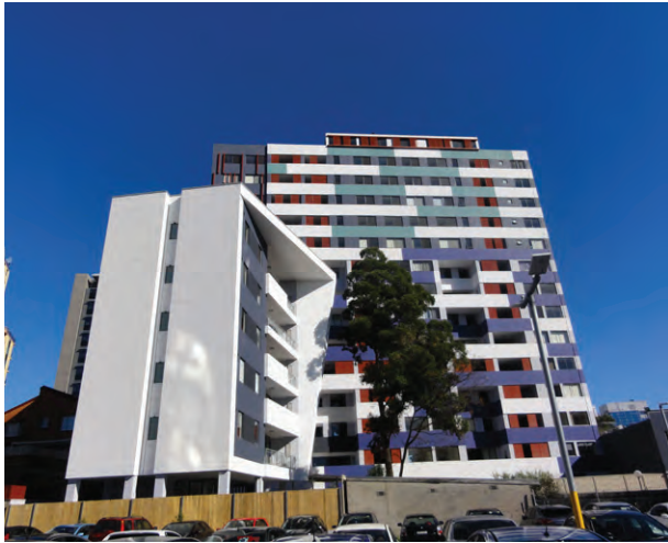
Recently developed 15 storey mixed use building - western boundary, fronting Charles Street
