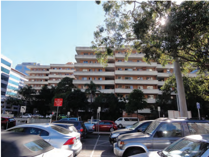
9 storey residential building to the north of the subject site on Macquarie Street
