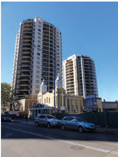
20 storey building at the southern cnr Hassall and Charles St
